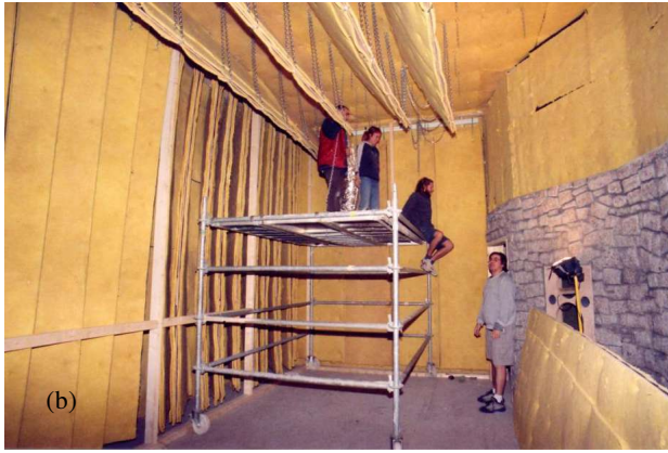
Figure 3. Room under construction, rear and with ceiling panels uncovered.
