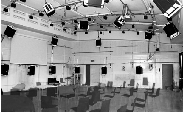
Figure 1. The IEM-CUBE is a concert room providing a 24-channel hemispherical Ambisonic system for 50 listeners.
