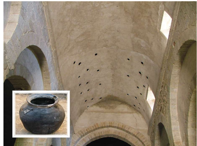
Figure 4. View of the vault in the nave of the church of Pommiers en Forez in Auvergne (France). Originally, each of the 29 holes corresponded to a pot. Only 27 are still in place, and 16 are unbroken. Bottom left: one of the pots removed from the roof and restored.
