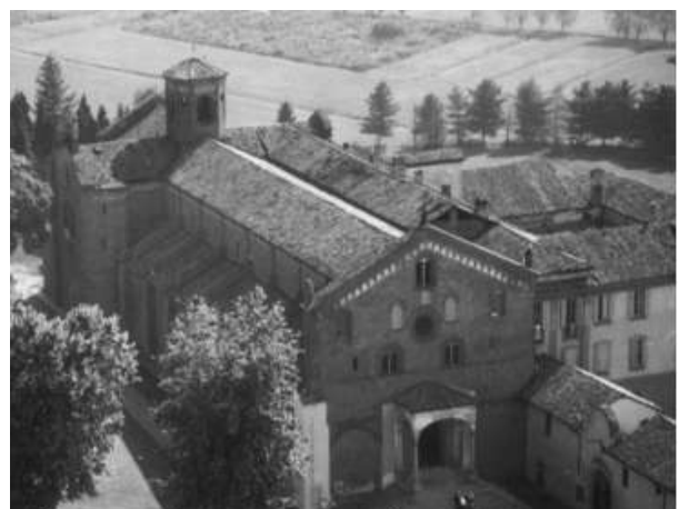
Figure 4: Morimondo – External view
