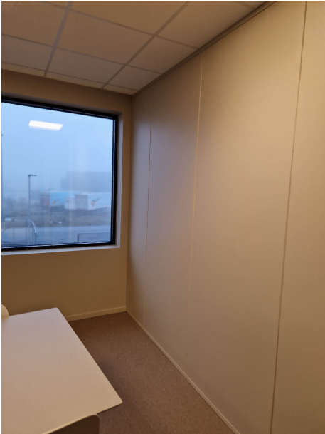
Figure 1. Office wall ended against ceiling plate.
