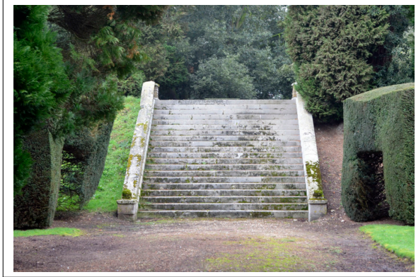
Figure 1. Steps at Terling Place.
