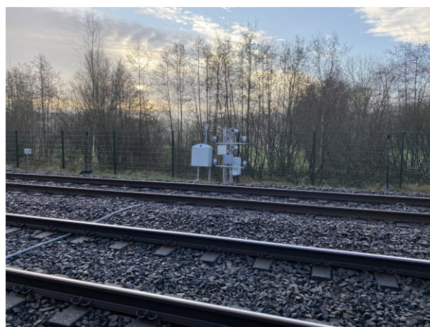
Figure 2. Onside installation of one of the two N-RSD systems for NEMO.
