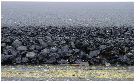
Figure 11. Side view of two-layer porous asphalt.
