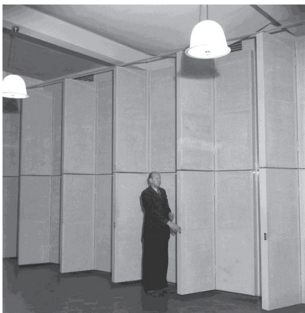
Figure 2. Paavo Arni presents the adjustable acoustics of the music studio of the Radio House of the Finnish Broadcasting Company in 1950. Source: Finnish Broadcasting Company Yle Archives.
