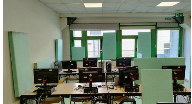
Figure 2. Internal view of the 135m 3 room with polyester fiber (PET) acoustic panels
