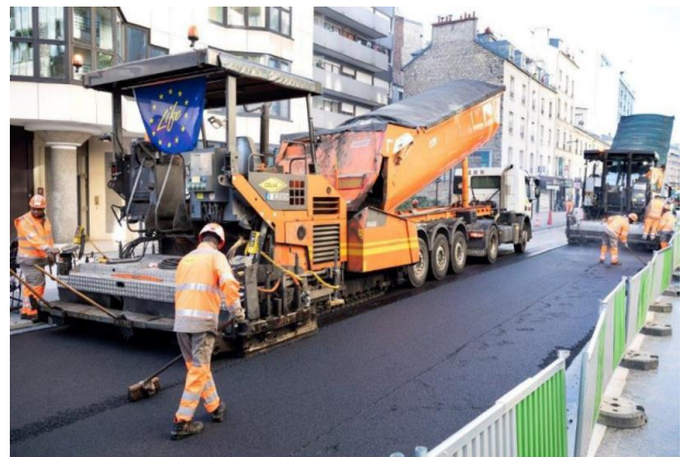
Figure 5. Frémicourt street with new asphalt mixes, October 2018.
