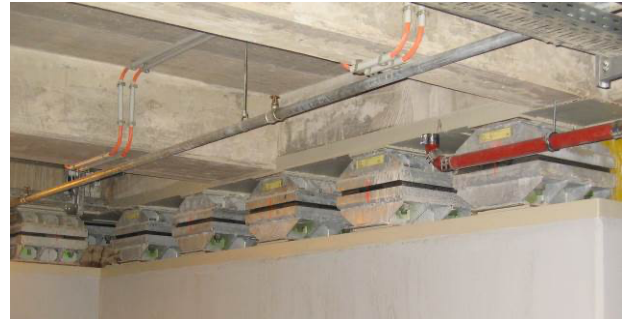
Figure 13. Elastic support elements between steel brackets (supplied by CDM, Belgium) under the Festival Theatre of the Palace of Arts. Designer P. Forián Szabó (2003-2005)
