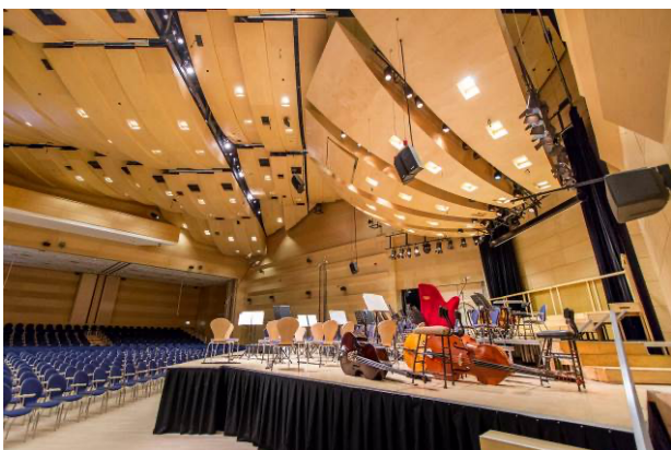
Figure 9. Digital room acoustics modification system, fabricated and installed by BEAG in the Kőlcsey Cultural Centre in Debrecen
