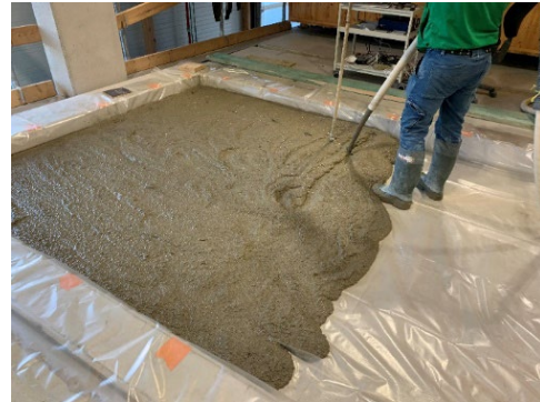
Figure 3. Application of the EPS thermal layer
