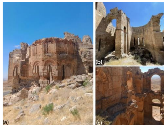
Figure 1. (a) An exterior view of Bell Church; (b) an interior view of the main church space (naos) with three apses; (c) the entrance hallway (narthex) of the church.
