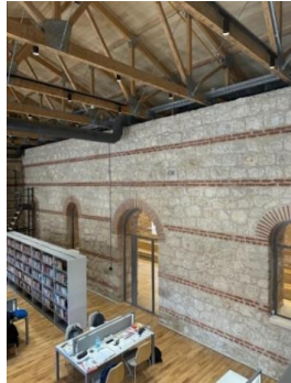
Figure 9. Rami Barrack stone masonry walls.
