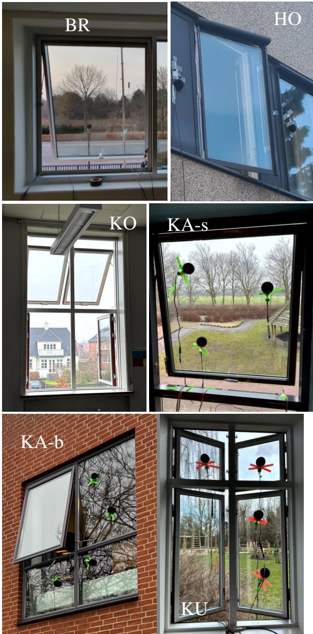
Figure 6. Photos of the field cases; KO includes both a top-guided and a side-opening window (sashes on the photos are opened more than 0.35 \text{ m}^2 ) and for KU both a combination of all windows open and a side-hung open window were measured.
