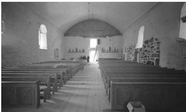
Figure 4. The nave of the church after the renovation was completed in 1962. (E. Lahtinen, Vapriikin kuva-arkisto, 1962)
