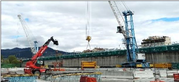
Figure 2. Cranes during earthmoving activity.
