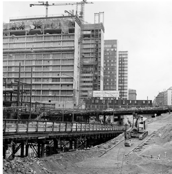
Figure 2. Building site 1961, typical multistory house with prefabricated elements [2].
