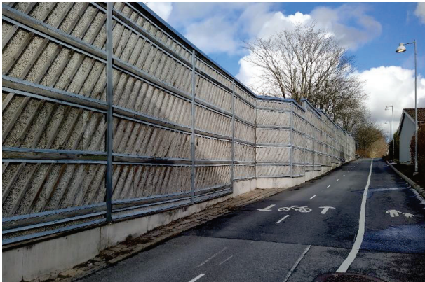
Figure 2. The Sävenäs timber noise barrier on the non-roadside.
