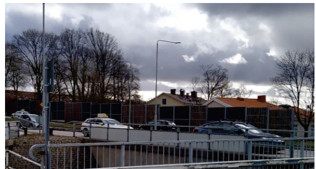
Figure 4. The noise barrier by the Torpa school.
