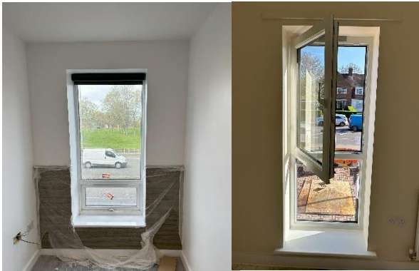
Photo 1: Site 1 Window Photo 2: Site 2 Window Open
