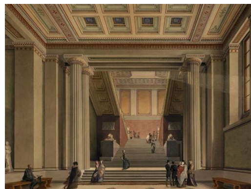
Figure 2. Illustration of Weston Hall (the main staircase) at the British Museum. Drawing, 1847 [10]
