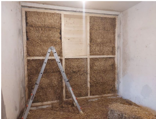
Figure 4. Wooden structure with straw filling
