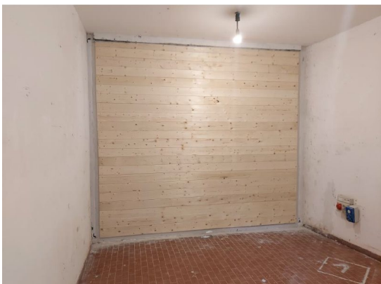
Figure 5. External side cladding with wooden planking
