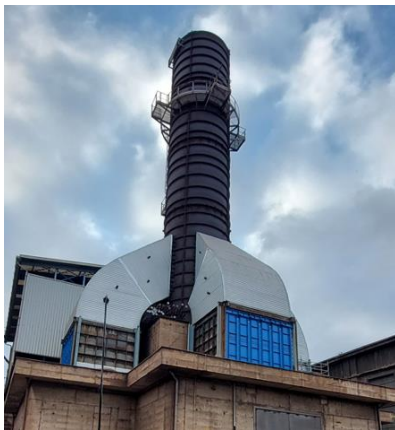
Figure 1. Chimney stack with three inlet ducts.
