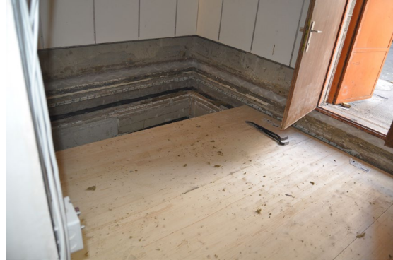
Figure 4. Installation of the bare timber frame ceiling in the test stand.
