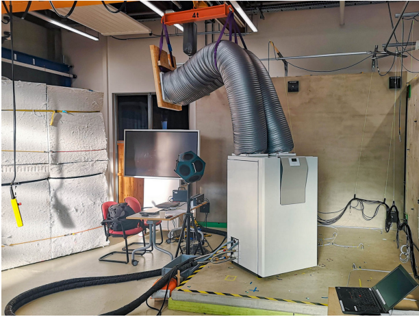
Figure 1: Heat pump with all required connections and piping for the operation mounted on a horizontal concrete reception plate.
