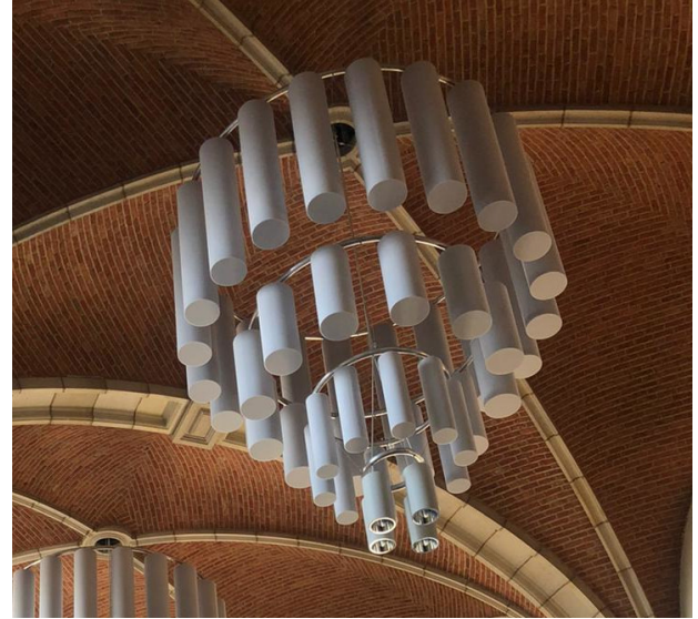
Figure 4. Final design of the sound absorbing chandelier, suspended from the ceiling of the Jubileumzaal.
