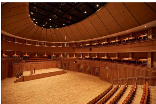
Figure 11. View of the oval sound transparent ceiling.
