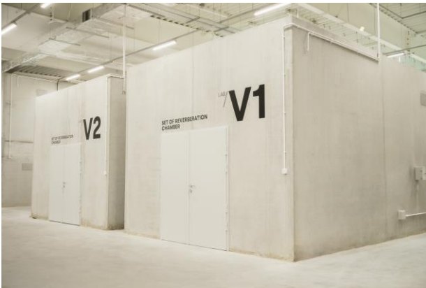
Figure 1. Two sets of reverberation chambers for isolation measurements at ARIC.
