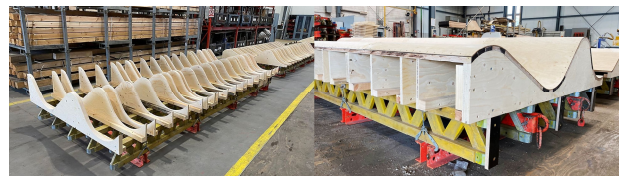
Figure 7. Creation of formwork for concrete works
