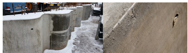
Figure 8. Verification of concrete quality
