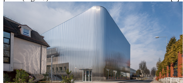
Figure 1. Jastrzębie Zdrój hall – exterior (finished)
