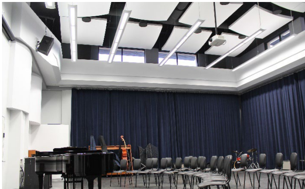
Figure 7. Photograph of the Band Rehearsal Room in University 1. The drapes can be retracted to expose large, curved sound diffusing wall planes below the acoustical shelf that surrounds the room at the upper level below the clerestory windows. The instructor commented that the acoustics are remarkable and the students enjoy playing in the room.
