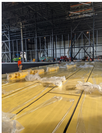
Figure 10. Sylomer mat during construction
