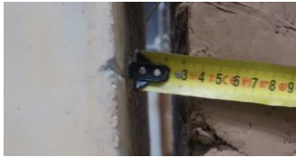
Figure 2. Peripheral shrinkage of an earth wall due to drying.
