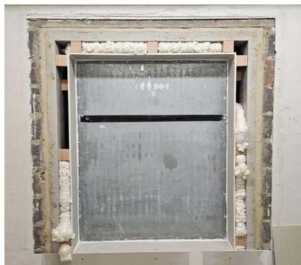
Figure 8. Example of a (partial) mounting using angle brackets on mounting blocks with a mounting gap of 8 cm and spray foamed interior reveals (interior side).
