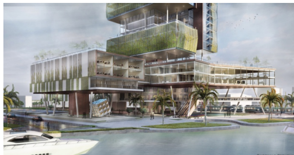
Figure 13. Sound diffusing building form with angular articulation, façade articulation at multiple scales, and layered panelized surfaces with moderate to good sound absorbing properties.
