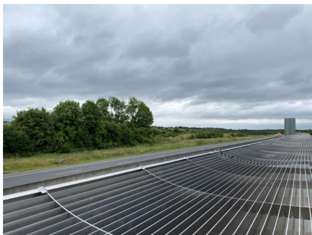
Figure 4. The WHIStop diffractor
