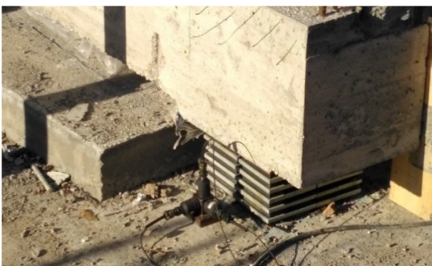
Figure 6. The isolation bearing, type Stravibase VHS, installed between the concrete distribution beams and the footings.
