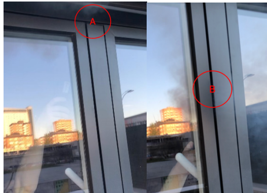
Figure 12. Visual identification of air leakage locations in House 2 using smoke detection
