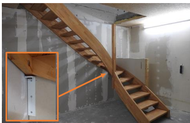
Figure 11. Wooden staircase with stringboard connected to the optimized wall construction with separated studs (Figure 9) and optimized corner support.
