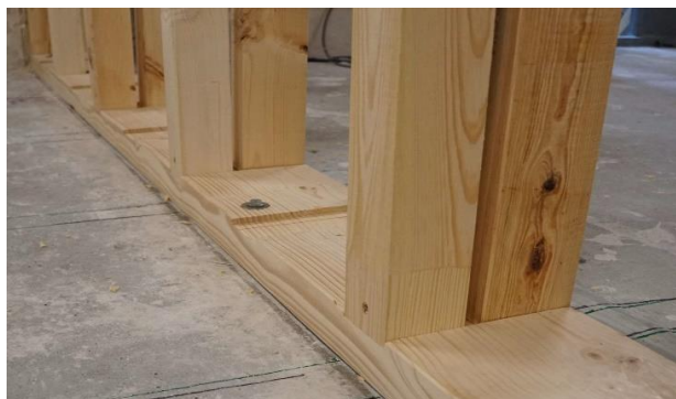
Figure 8. Timber stud wall with separated studs and continuous sill and frame.
