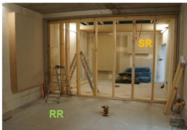
Figure 2. Frame construction of the timber stud wall.
