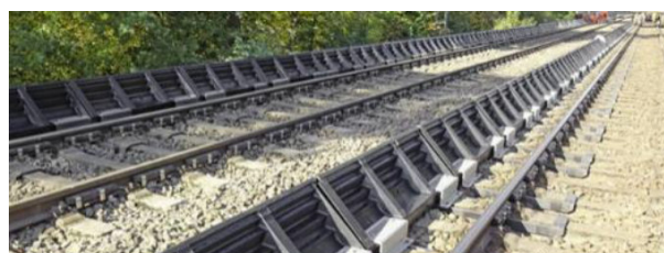
Figure 1. Example of a low-height noise barrier (LHNB).
