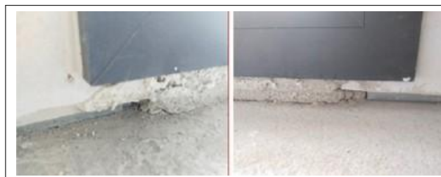
Figure 7. Acoustic bridges in critical room.
