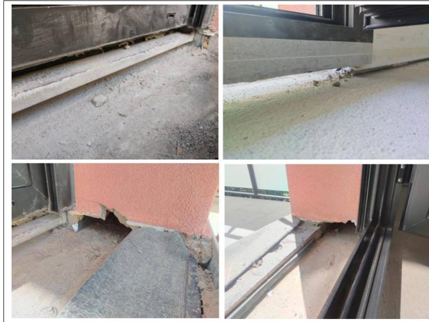
Figure 8. Removing the acoustic bridges before the final assessment.
