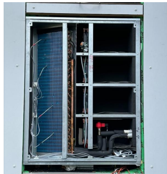
Figure 2. Outdoor unit of a façade-integrated mini split air-to-water heat pump for domestic hot water installed at the University of Innsbruck.
