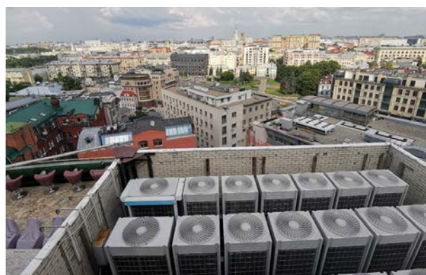
Figure 1. Dry coolers on the roof.
