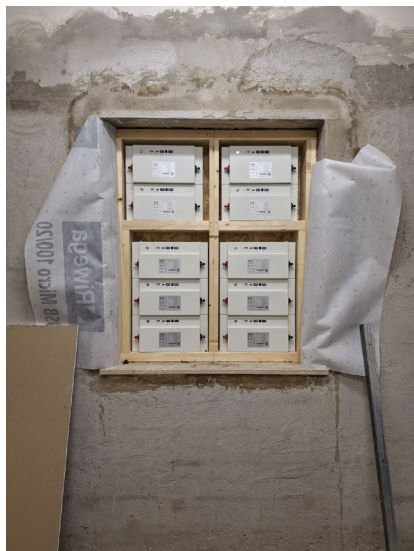
Figure 7. View of the sample with storage devices, before internal finishing.
