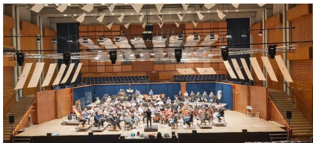
Figure 5. Views towards the stage in CN with tilted reflectors suspended over both sides of the stage.
