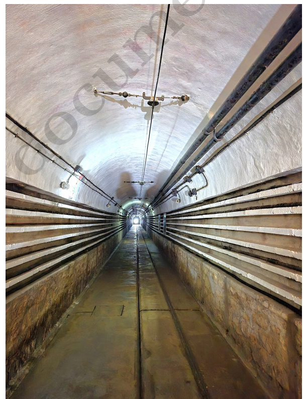
Figure 2: 300 m long tunnel.
