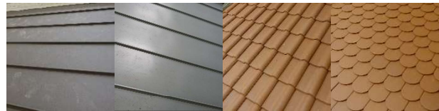
Figure 3: Roof claddings investigated, from left to right: aluminium sheet, zinc sheet, tile 1 (sliding tile), tile 2 (beaver-tail tile)
