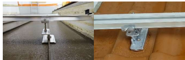
Figure 5: PV substructure — left: on aluminium sheet cladding; right: on tile cladding
