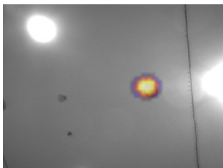
Figure 5. Illustration of one of the loudspeakers of the PAVA system in a shopping centre.
