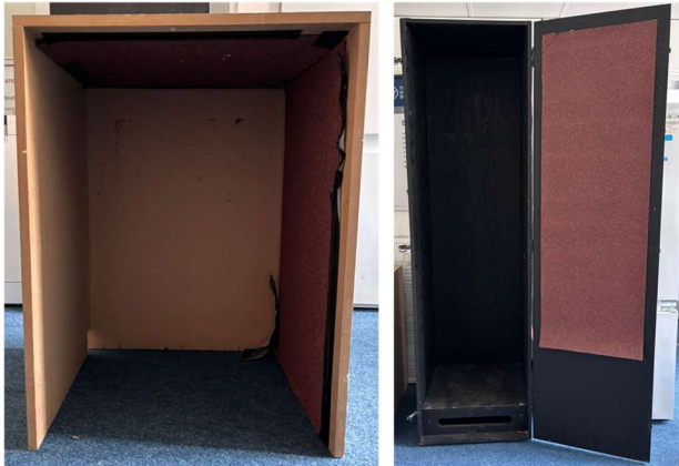
Figure 1. Investigated built-in kitchen enclosures: dishwasher enclosure (left) and refrigerator enclosure (right).
