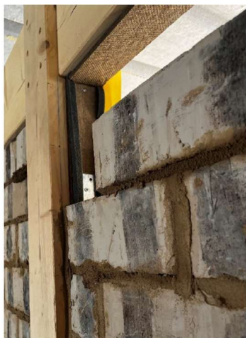
Figure 5. Wall D separated with wood post at the centre.
