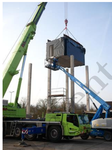
Figure 5. Lifting a room module into the primary structure of the mock-up using a mobile crane.
