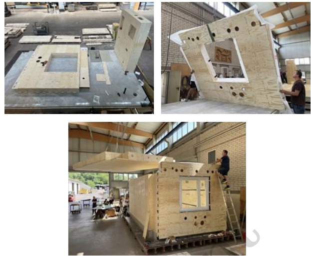
Figure 2. Construction of the room module prototype - components on the base plate (top left), erecting the external wall with the window opening (top right), fitting the ceiling (bottom).
