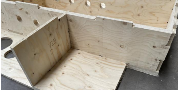
Figure 1. Interlocking system made from 18 mm thick plywood panels for constructing the wall and ceiling components.
